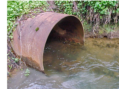
Before – A 4-foot round steel culvert at Mosquito Creek on US 101.
