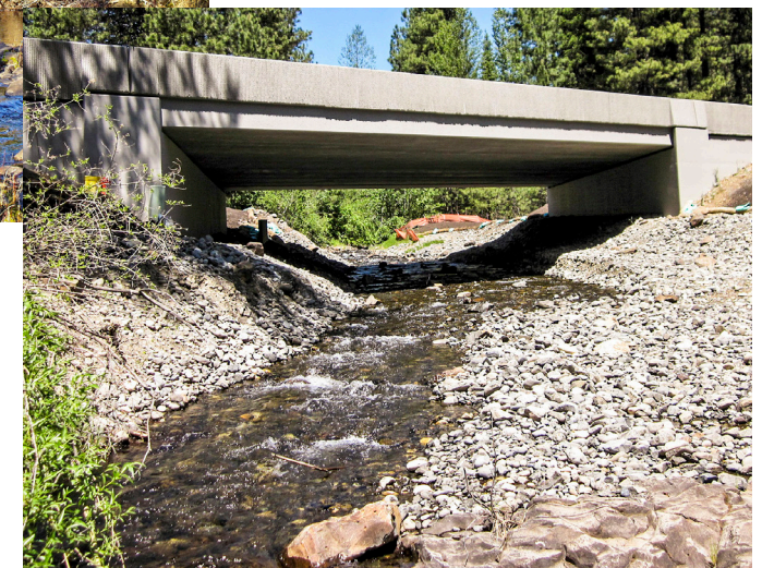
After – The 11 foot culvert was replaced with a 65 foot bridge at Butler Creek at milepost 21.35 in 2012 for $3.5 million.
